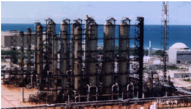
Figure 2.6. The Ontario Hydro International Bruce Point Heavy Water Plant had the capacity to produce 800 tons of per year. It was shut down in 1997. Eight plants of this size could supply enough heavy water to generate all of the energy now consumed in the world.
