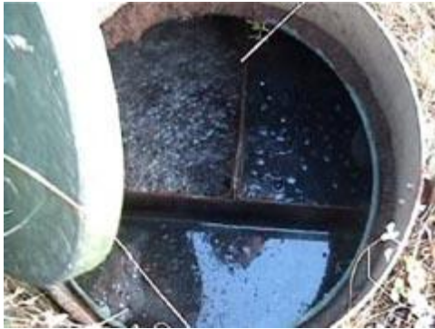
Grease-trap/septic tank + sandfilter + sample/pump pit
