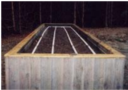
Laying the greywater irrigation pipes
