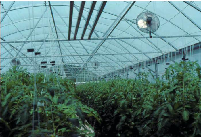
Figure 27. Horizontal air-flow fan for circulating air in greenhouse.
