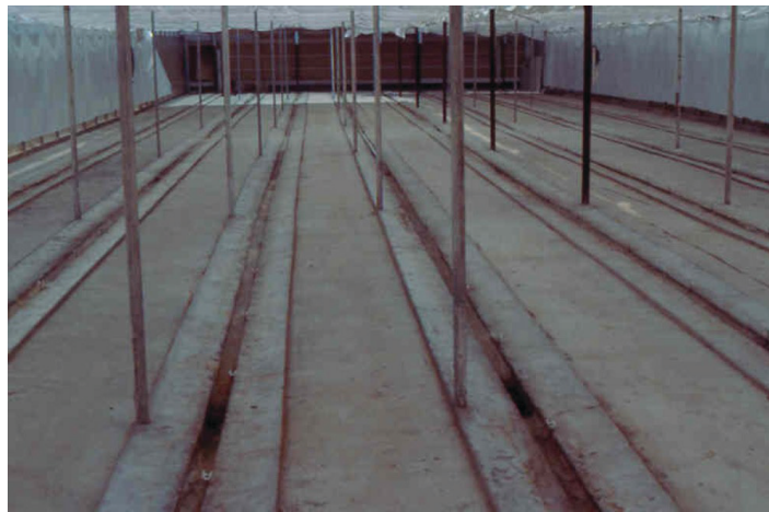
Figure 10. Inclined concrete leachate troughs on which growing bags are placed.
