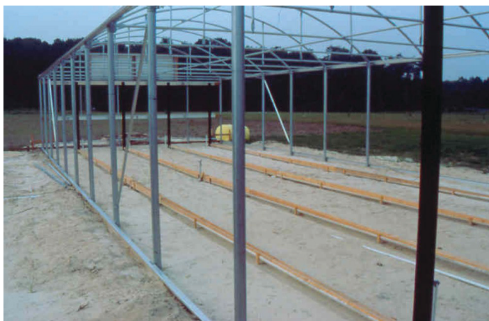
Figure 25. Installing greenhouse floor with leachate collection system.
