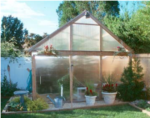
The author built this simple 8x12' greenhouse in his yard in just a few weekends and for less than $1200 in lumber and GE Thermoclear glazing.
