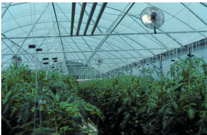
Figure 20. Horizontal air-flow fans.
