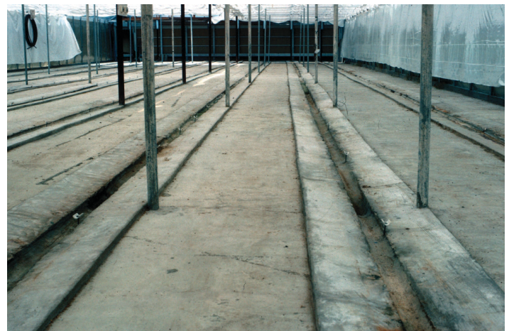
Figure 16. Concrete slanted pads for drainage leachate.
