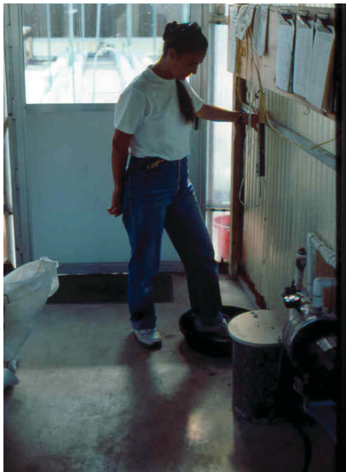
Figure 11. Entrance air-lock porch provides space for foot bath for sanitation purposes.
