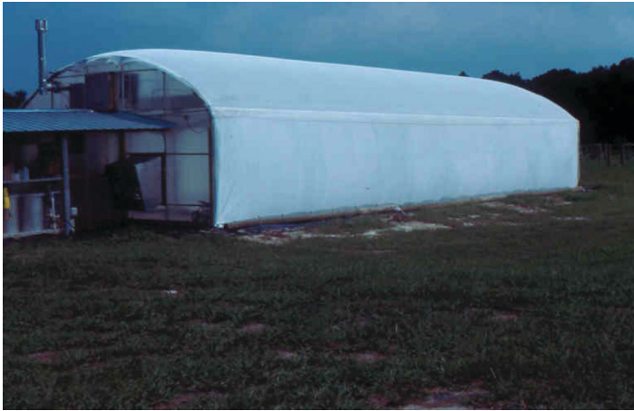
Figure 4. Small single-unit greenhouse.
