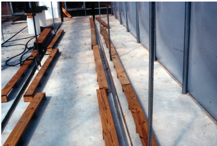
Figure 18. Drainage troughs created by pouring concrete floor around wooden forms and then removing forms, leaving behind troughs. Wooden benches also shown in photo.
