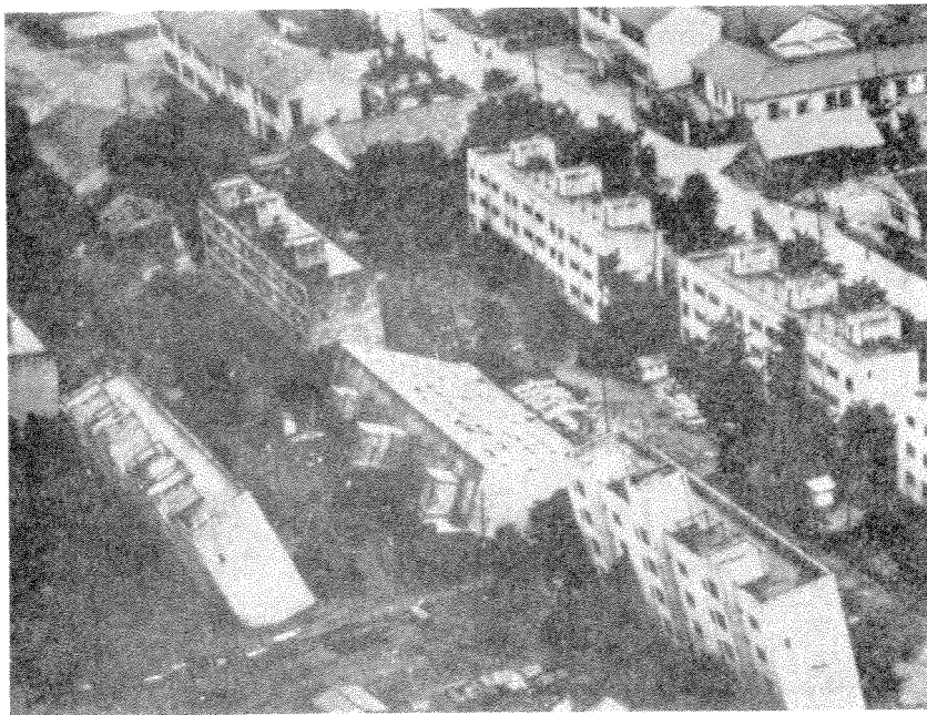
TILTED APARTMENT HOUSE AFTER EARTHQUAKE IN NIIGATA, JAPAN
