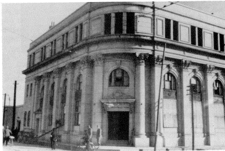
Geibi Bank Co. building after attack on Hiroshima
