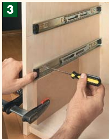
◀ Using a Spacer. Rest the drawer slide on the spacer and install the screws. After transferring the mark for the lower drawer slide to the spacer, cut it to length and repeat the process.
