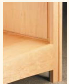
▲ ... but their inside faces have been rabbeted so that the frames and panels are flush inside the case.
