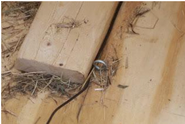
Setting up the wire for a new bale.
