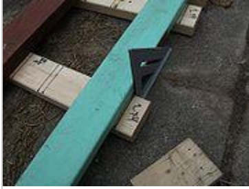
Fig 2a: Using a square & Marking Wood
