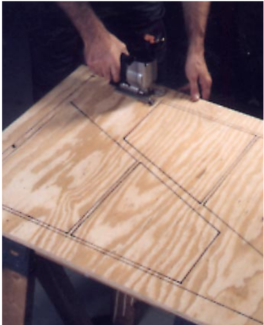
A handheld jigsaw makes quick work of cutting out parts C, D, and E. Cut close to the line then sand to it.
